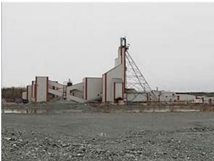
Surface plant of the Sleeping Giant mine
