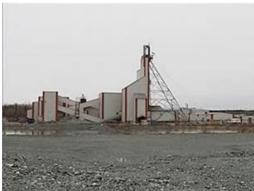
Surface plant of the Sleeping Giant mine
