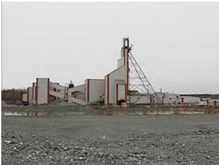
Surface plant of the Sleeping Giant mine
